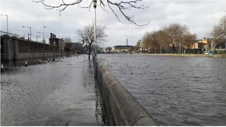
Figure 4: Flooding at Victoria Quay in January 2014
