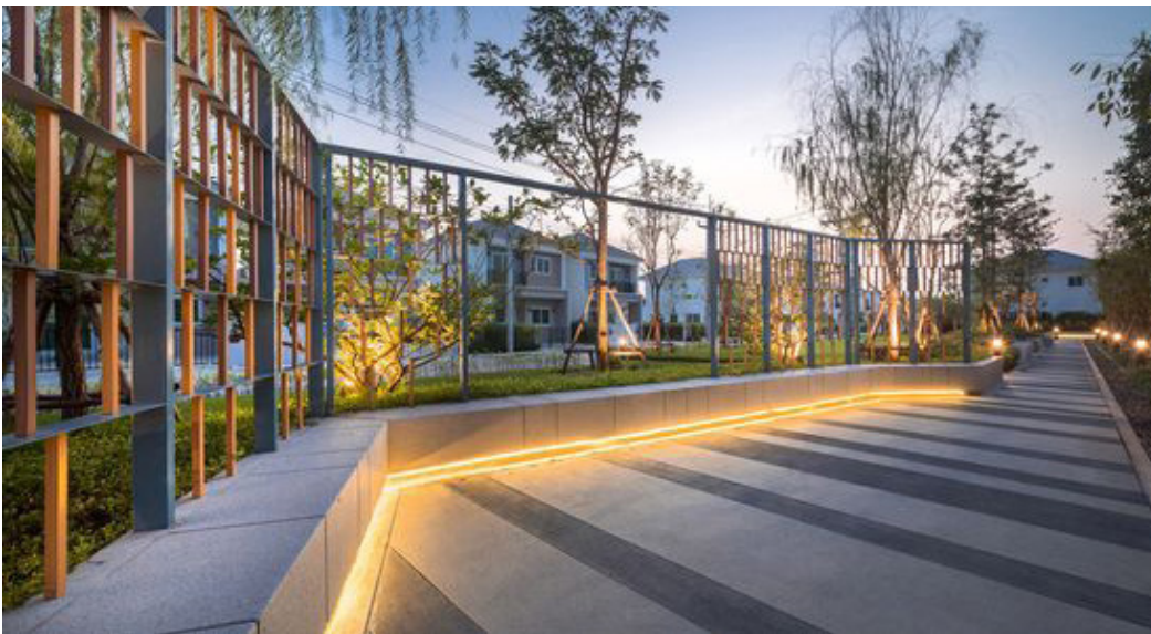
Pre cast concrete planters with lighting strip
