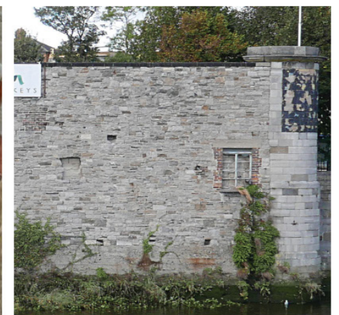
Quay Wall and Turret
