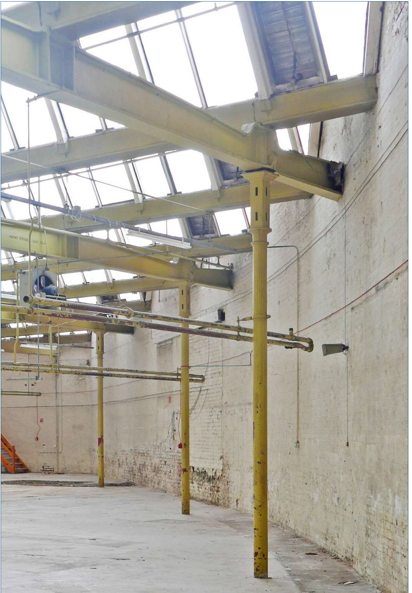
View looking at the inside of the curving wall to Parkgate Street at the north east of the warehouse. This view shows several main beams cut short as they enter the wall.
