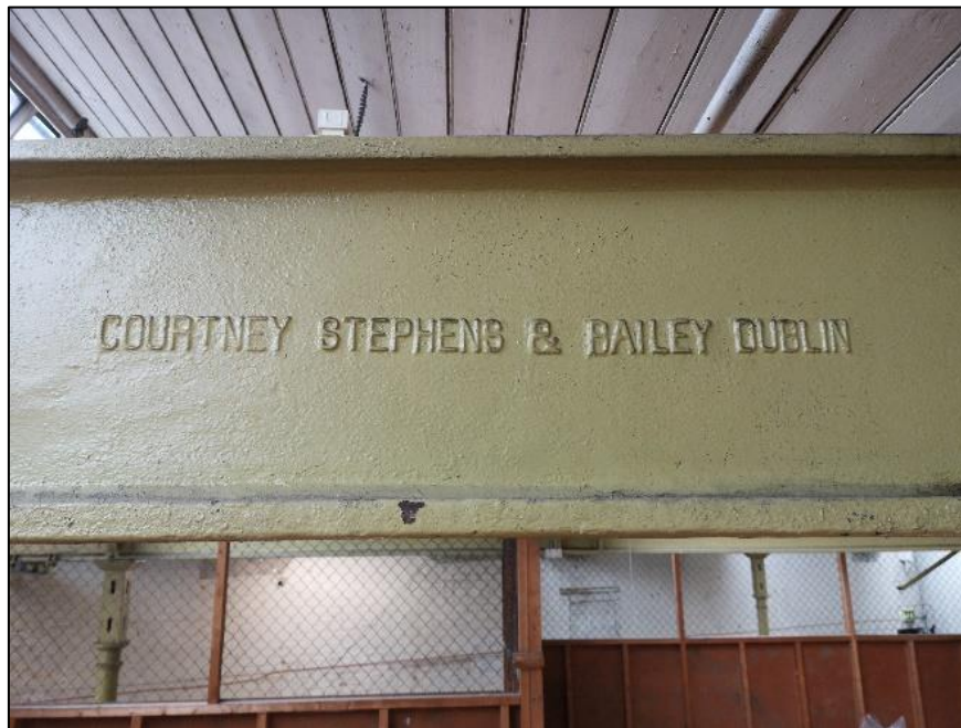
Plate 2 An example of Ironwork within the factory from an engineering partnership formed in 1865
