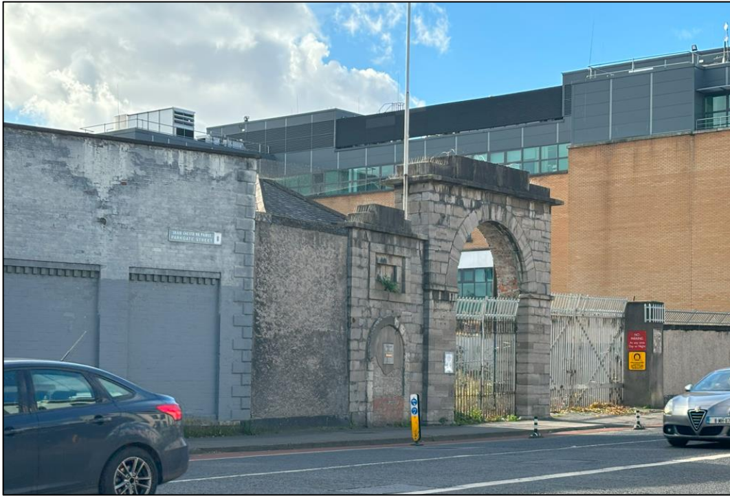
Plate 1 Original entrance gate to east of modern gates on Parkgate Street, facing SW
