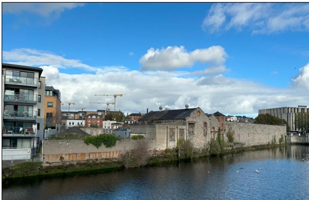
Plate 8 View of riverside wall, turret and buildings from the south side of the River Liffey
