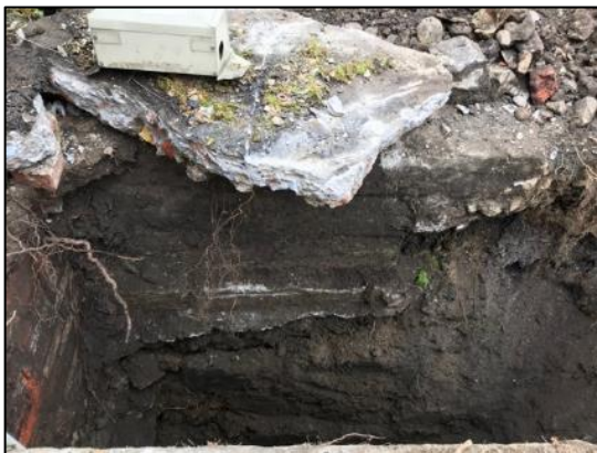
Plate 1 Concrete wall supports
