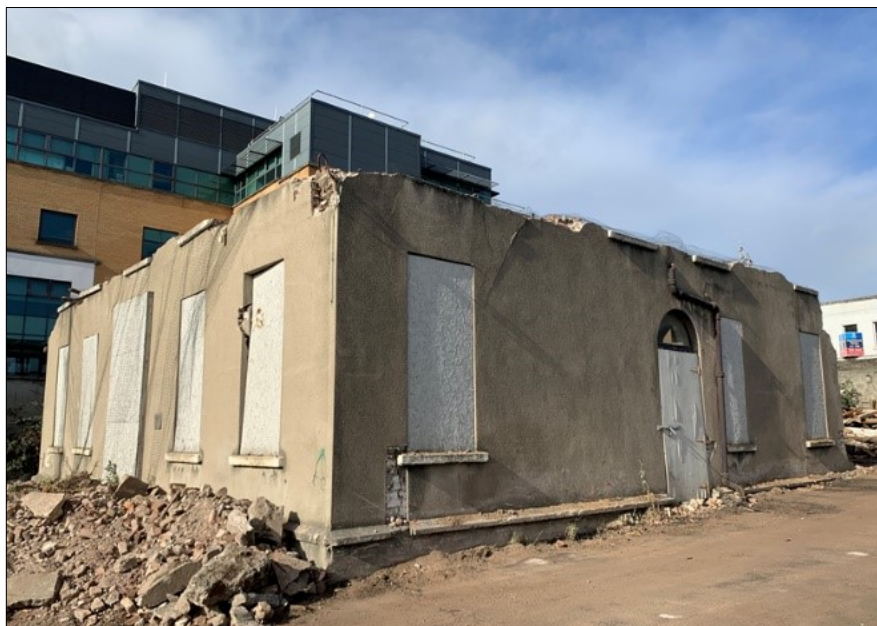
Plate 2 Parkgate House post demolition of upper floors
