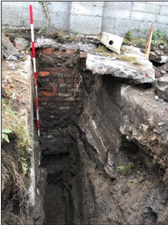
Plate 3 Inner face of quay wall
