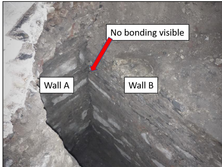
Plate 20 Test Pit 8 showing that Wall A and B are not tied in, view to northwest
