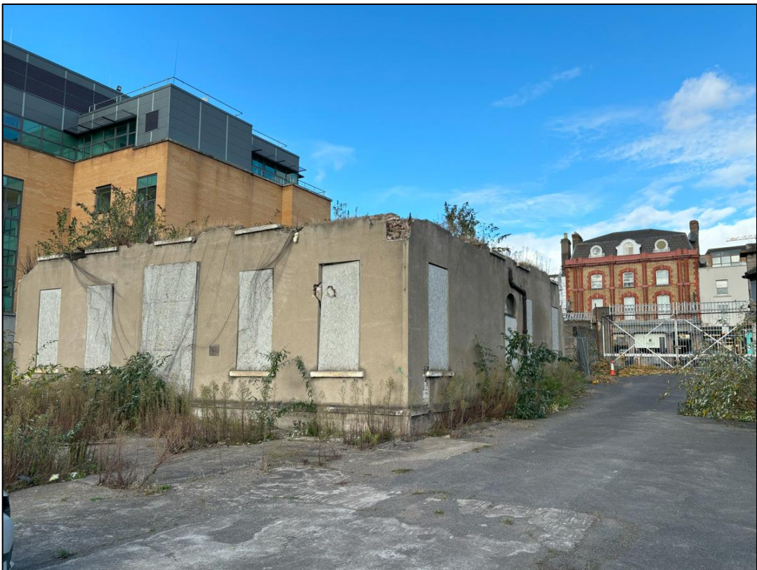
Plate 4 Part-demolished 19 th century house, facing NE
