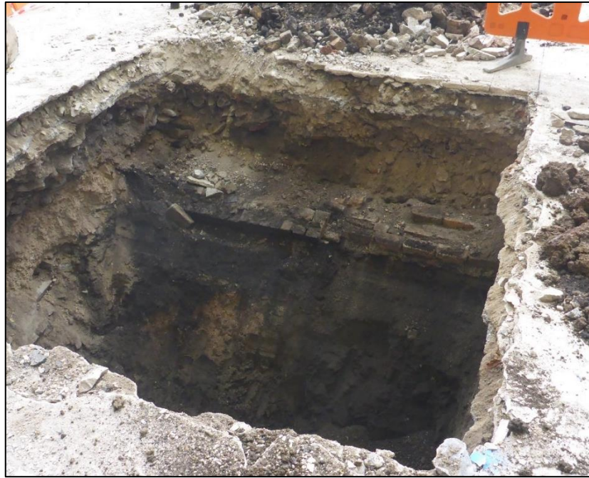
Plate 9 Test Pit 2 showing wall, view to northwest
