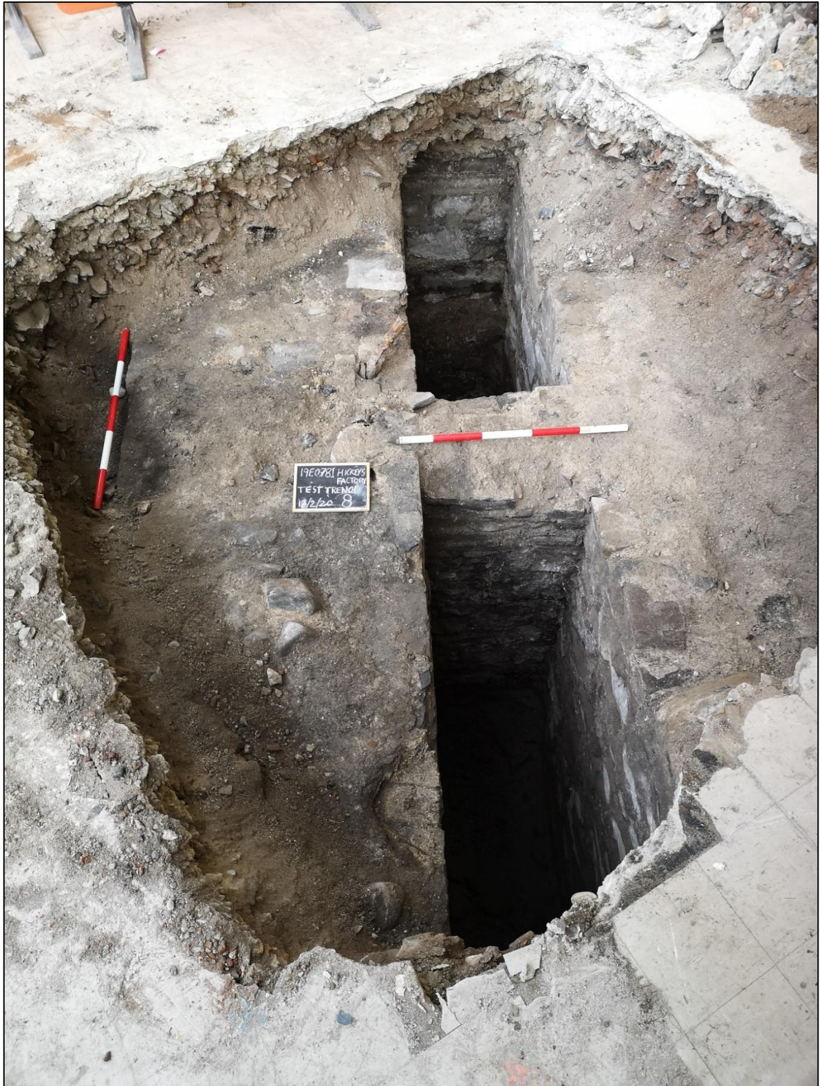
Plate 19 Test Pit 8 looking southeast showing the possible limestone flue structure, view to southeast
