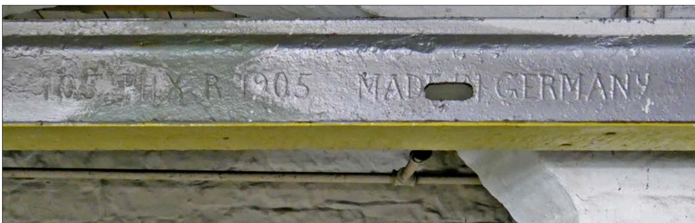
'105 PHX R 1905 Made in Germany' marked on a length of tram track forming part of a mezzanine structure near the south wall of the Warehouse. It is possible that the mezzanine was built when the building was a munitions factory, making shells to fire at the Germans.
