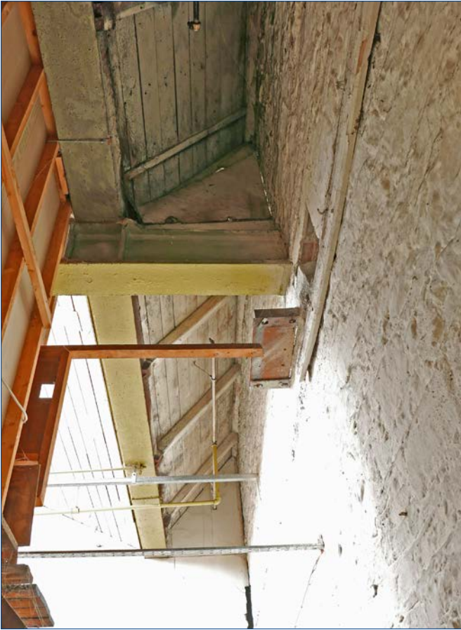
Inside of the Riverside Stone Wall, looking east and upwards near the east end of the wall. At the east end of the warehouse, two cast iron roof beams continue to the Riverside Stone Wall. The rest of the beams do not
