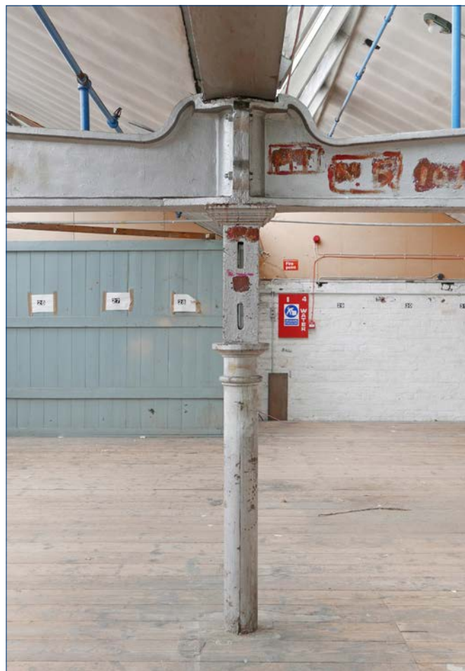
Detail at the head of a column showing the meeting of two roof beams and the cast iron gutter beam above.
