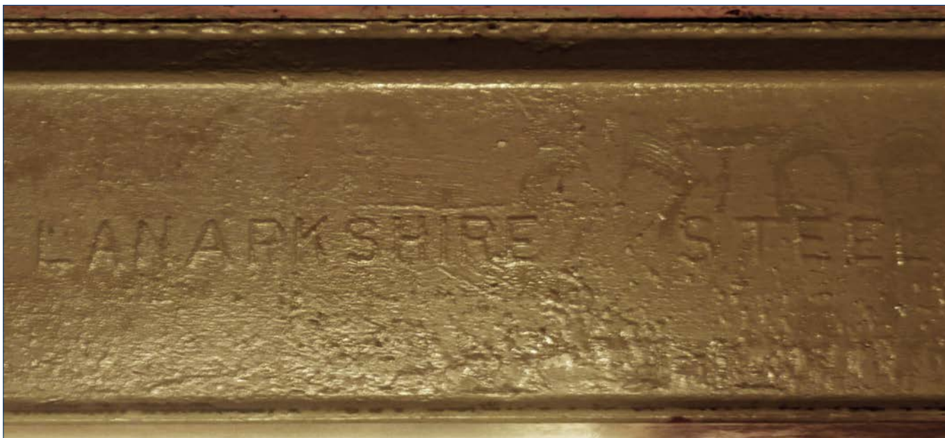
The name 'Lanarkshire Steel' marked on a rolled steel joist near the western side of the Warehouse.
