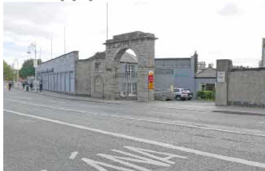
Parkgate Street - Existing Stone Arch
